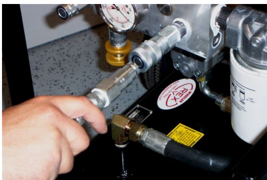
Lines being attached to the Power Pack
